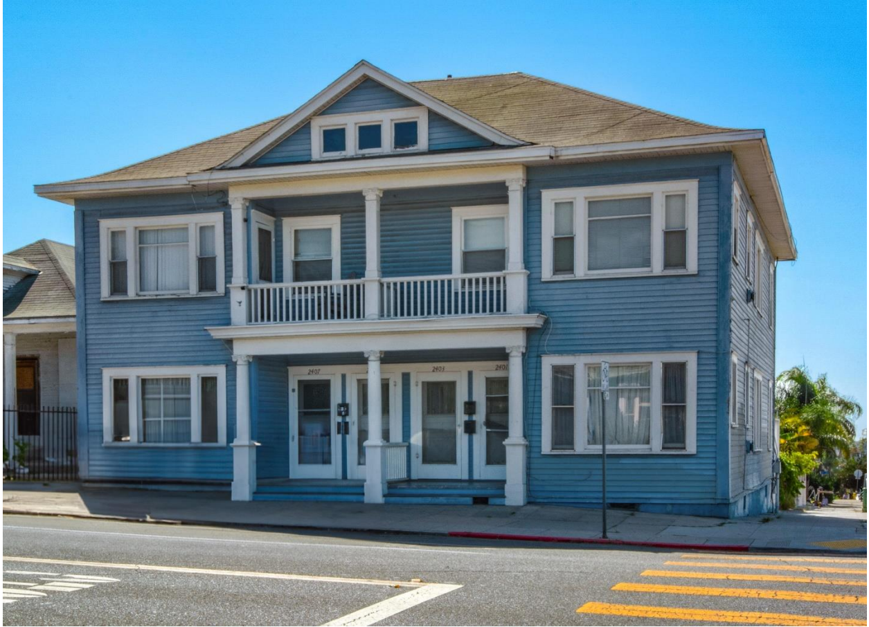
Island Avenue Entry
