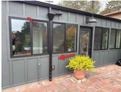
North Backyard Gutter Downspout
