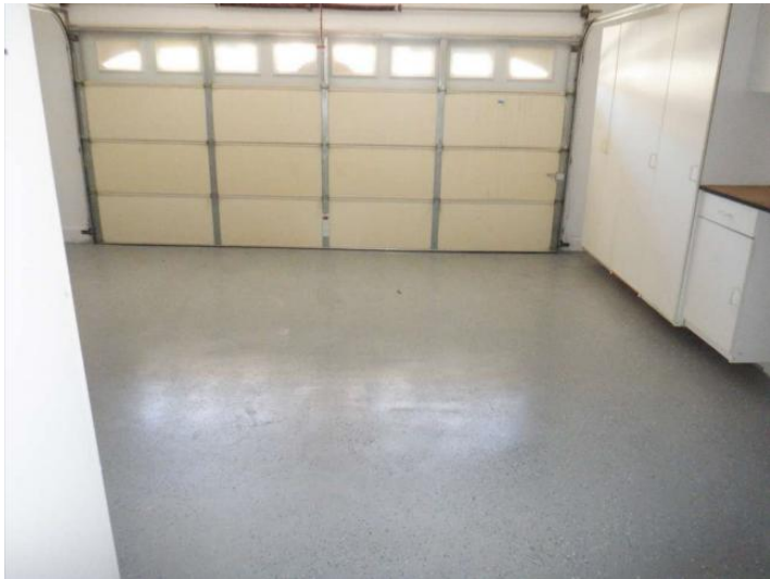
Garage new Epoxy floors
