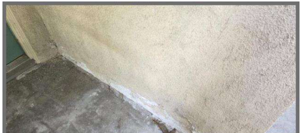
peeling/ moisture deterioration
