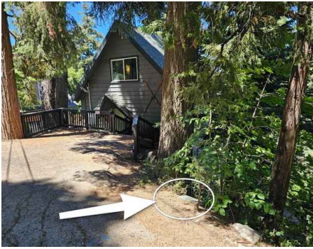
Water Meter Box
