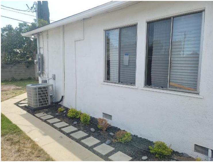
Electrical Information / Sub Panel 1 Labels, Location Pullbacks and 360 views
