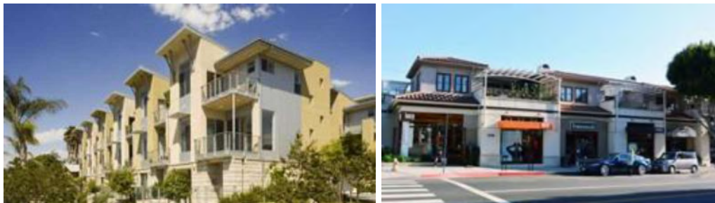
ARCHITECTURAL PROJECTIONS AND RECESSIONS PROVIDE INTEREST AND A HUMAN SCALE TO BUILDING FACADES.
