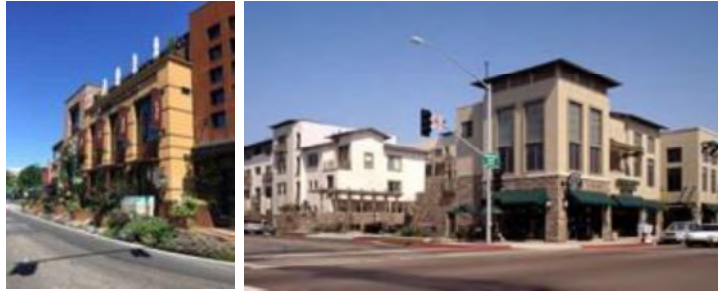
VERTICAL ARTICULATION CAN BE ACHIEVED BY VARIATIONS IN HEIGHT WITHIN A BUILDING’S MASSING.
