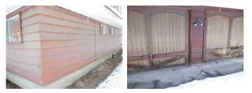
• One section of the wood siding on the side of the garage has a cut out that should be repaired
