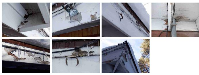
· Wood damage noted on some section of the eaves- confirm with termite control co
