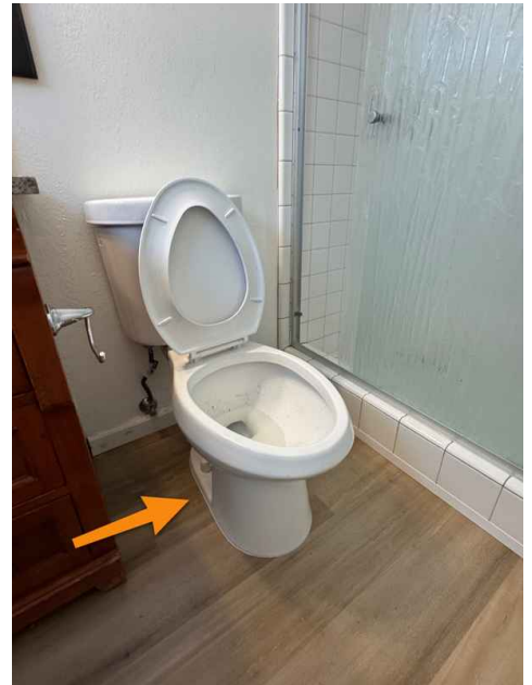
Primary Bathroom Toilet
