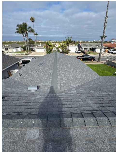
Front, Garage Roof
