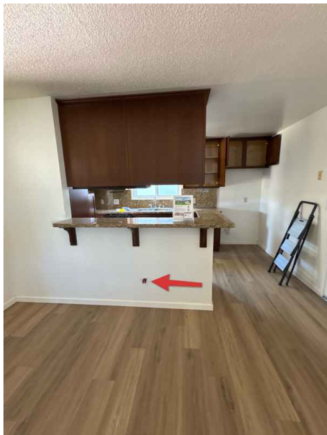
Example noted at Kitchen
