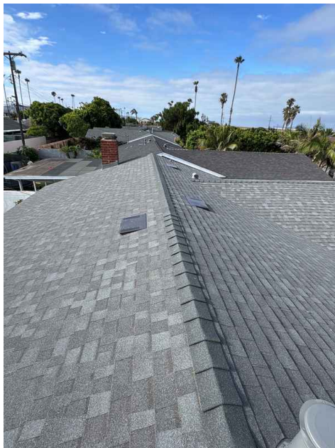
Right Side Roof
