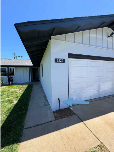
Example noted at Front of Home
