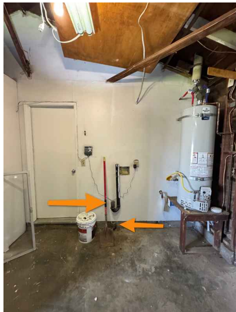
Garage Rear, Laundry Area
