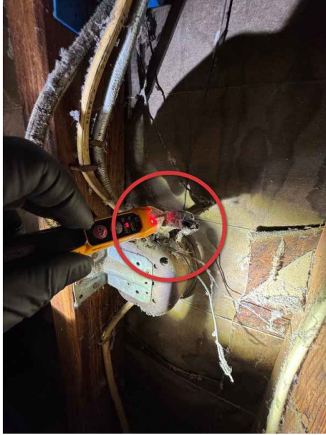
Example noted, wire appeared powered
