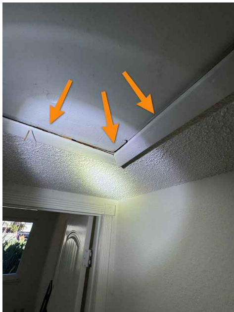
Attic hatch, Hallway
