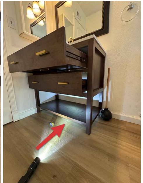
Example noted at Hall Bathroom, Below Sink
