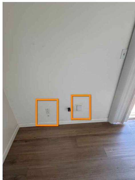
Example noted at Living Room
