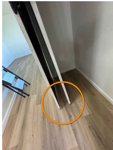
Primary Bedroom Closet
