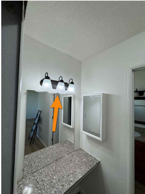
Example noted at Primary Bedroom
