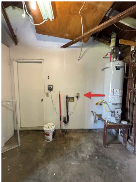
Example noted at Garage Laundry Area
