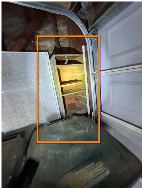
Example noted at Garage, Left Side facing outwards
