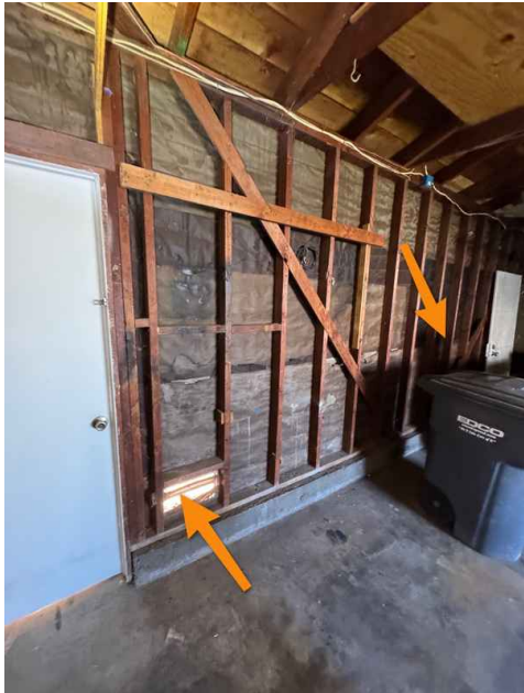
Garage, Left Side facing outwards
