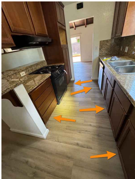
Example noted at Kitchen
