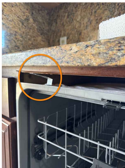
Unit not secured
