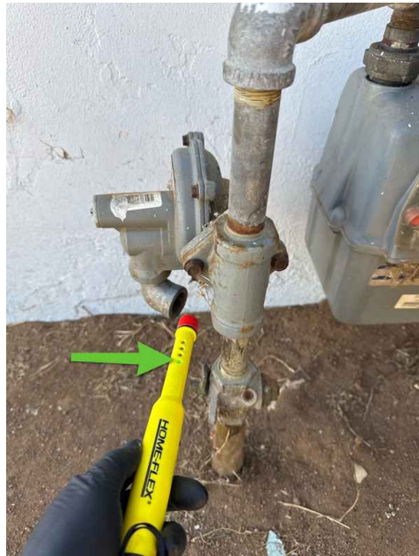
No gas leak detected at time of inspection
