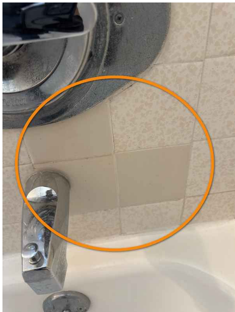
Example of Repairs noted at Hall Bathroom Shower
