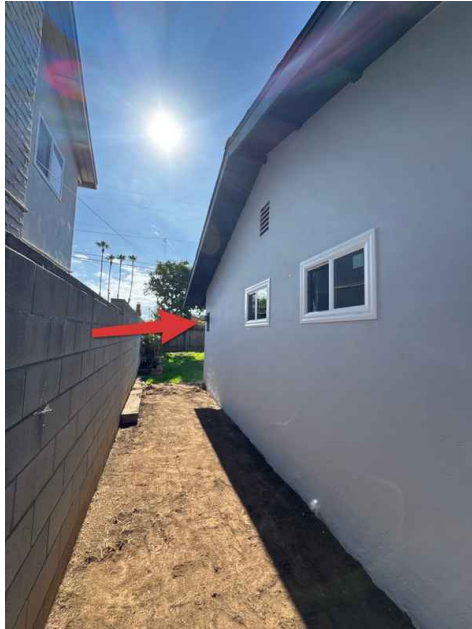
Main Panel, Left Side of Home
