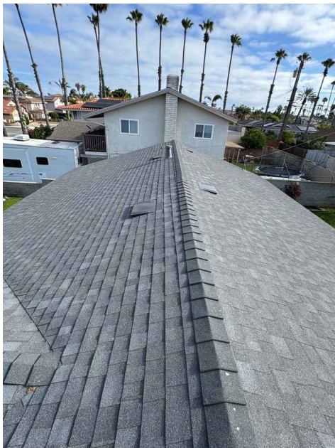
Left Side Roof
