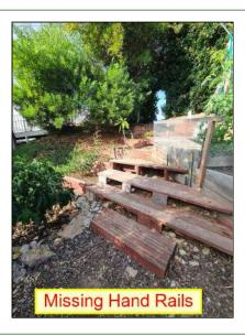
(2) Trip Hazards. There were areas that contained raised items, which extended above the walkway's surface. These areas may pose as trip hazards. This was noted at the front yard stairs. It is recommended that adjustments be made to create a smooth walking surface at these locations or a large obstacle be placed in front or over these areas.
