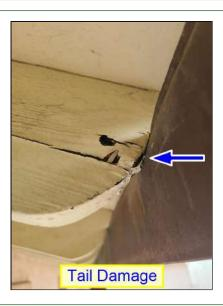
(3) Eave Damage. There was some wood damage at some of the eaves at the front of the property. It is recommended that you read your termite report thoroughly and that any damaged wood be repaired or replaced by a licensed contractor if needed.
