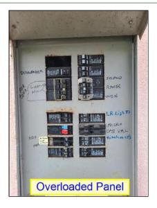
(6) Breakers Not Properly Labeled. The breakers in the main panel are not all labeled for individual use or are improperly labeled. It is recommended that each breaker be labeled for its correct use for easy identification. Recommend that an electrician correctly identify and label each breaker for its use.
