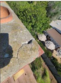
(4) Low Chimney. Chimneys should terminate 3 feet above the roof and be 2 feet above any part of the building within ten a foot radius. Currently this chimney meets the roof clearance, however it does not meet the 10 foot radius requirements. Currently the top of this chimney is less than three feet from the roof. This is noted for your information and should be corrected by a licensed contractor.
