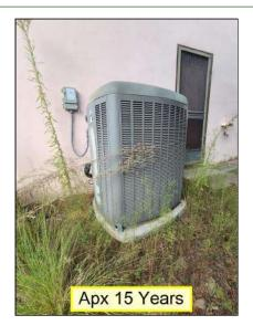
(2) Underpinning Noted. There was some underpinning noted at the dA/C pad. There are some areas of soil erosion at some of the exterior pad. Underpinning occurs when the soil is removed from the underside of a structure, weakening the support. This can cause the unit to move and become unlevel. It is recommended that these areas be further evaluated and repaired as needed.
