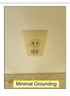
(3) Improper Conversion- Ungrounded. Many of the electrical outlets in the rooms are not grounded, and were originally installed with two-pronged (ungrounded type) outlets. For convenience purposes, most of these
