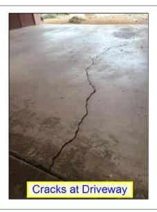
(3) Poor Drainage. The base of the driveway did not have good drainage. It is recommended that drainage be provided at the base of the driveway.
