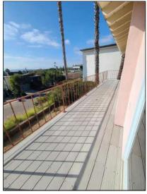
(2) Wide Spacing. The spindles at the exterior railings are currently spaced greater than 4 inches. Although this may have been standard at the time this was built, is recommended for today's standards, that the spacing of these spindles be no greater than 4 inches. This is a safety measure to help ensure that a child cannot slip through this area. It is recommended that you add a screen or more balusters at this location.
