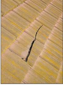
(3) Loose Tiles. There was an unsecured or loose tile noted at the roof. Loose or unsecured tiles can slip or move, exposing the roofing felt and increasing the risk of damage and roof leaks. It is recommended that the roof be further evaluated for possible loose tiles and that all tiles be properly secured by a licensed roofing contractor.
