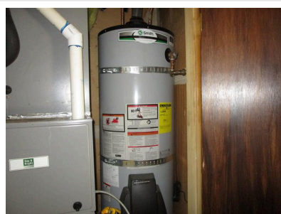
7.6 Item 1(Picture) family room closet
