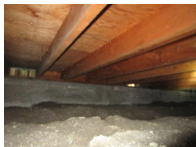
4.6 Item 1(Picture) south side
