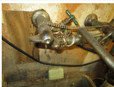
7.7 Item 1(Picture) garage sink
