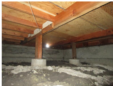
4.6 Item 14(Picture) rear addition
