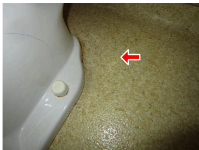
9.6 Item 1(Picture) master bathroom
