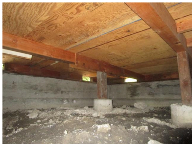
4.6 Item 13(Picture) rear addition
