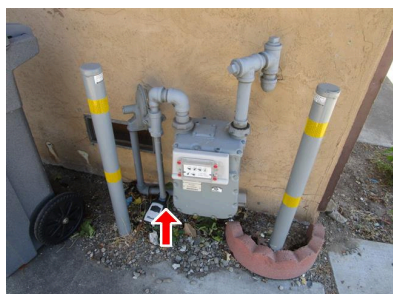
1.2 Item 1(Picture) side of garage
