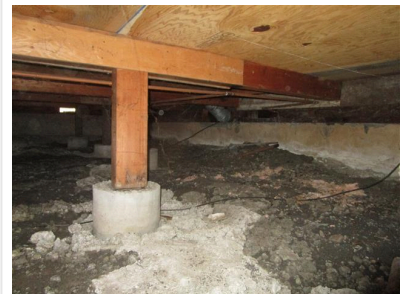
4.6 Item 15(Picture) rear addition
