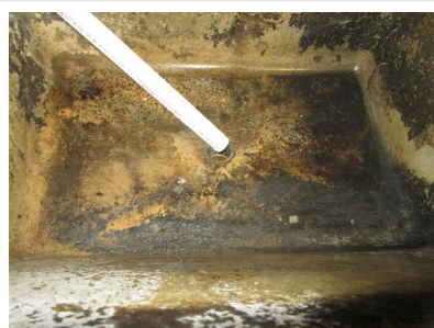
7.8 Item 1(Picture) garage sink
