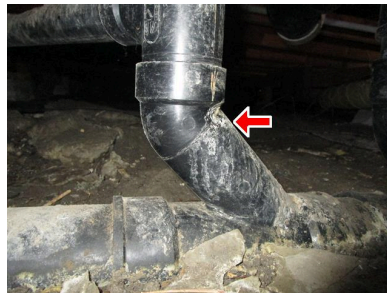
7.3 Item 2(Picture) hall bathroom
