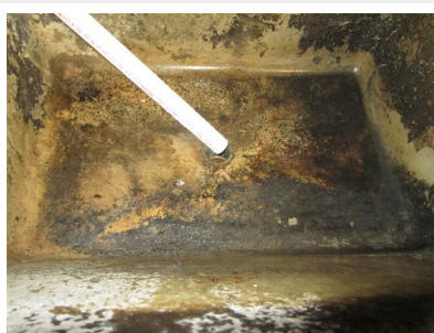
7.8 Item 1(Picture) garage sink
