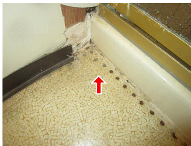
9.6 Item 2(Picture) guest bathroom
