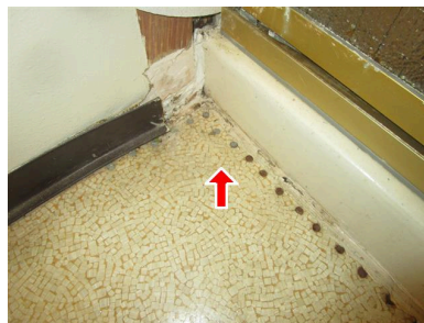
9.6 Item 2(Picture) guest bathroom
