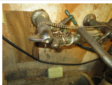
7.7 Item 1(Picture) garage sink
