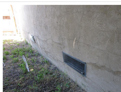
3.5 Item 3(Picture) south side
