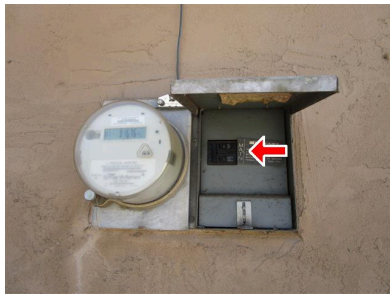
1.4 Item 1(Picture) side of garage
