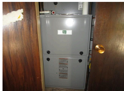
8.0 Item 1(Picture) family room closet
