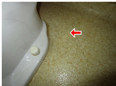
9.6 Item 1(Picture) master bathroom
