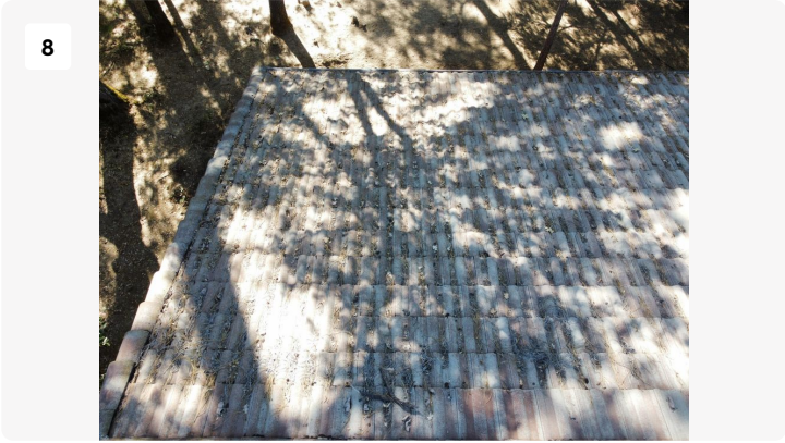
Project: 21919 Fallview Dr, Sonora, CA 95370, USA Date: Aug 14, 2026, 3:57 PM Creator: Steven Alvarez Tags: Roof Debris - Clean
