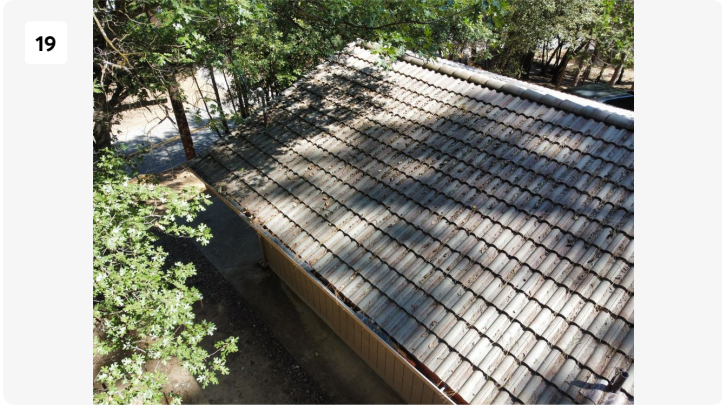
Project: 21919 Fallview Dr, Sonora, CA 95370, USA Date: Aug 14, 2026, 3:58 PM Creator: Steven Alvarez Tags: Discontinued - Roma Tile
