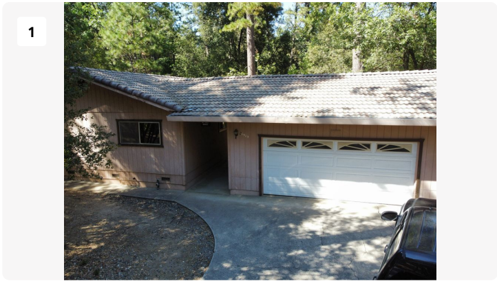
Project: 21919 Fallview Dr, Sonora, CA 95370, USA Date: Aug 14, 2026, 3:57 PM Creator: Steven Alvarez Tags: Discontinued - Roma Tile
