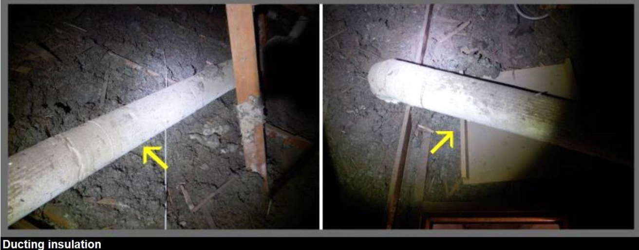
Ducting insulation
