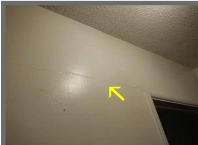
Cracks & rough patching
