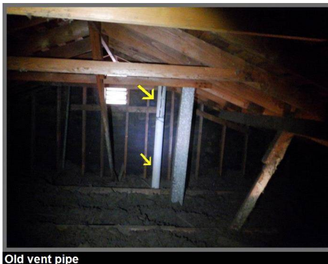
Old vent pipe
