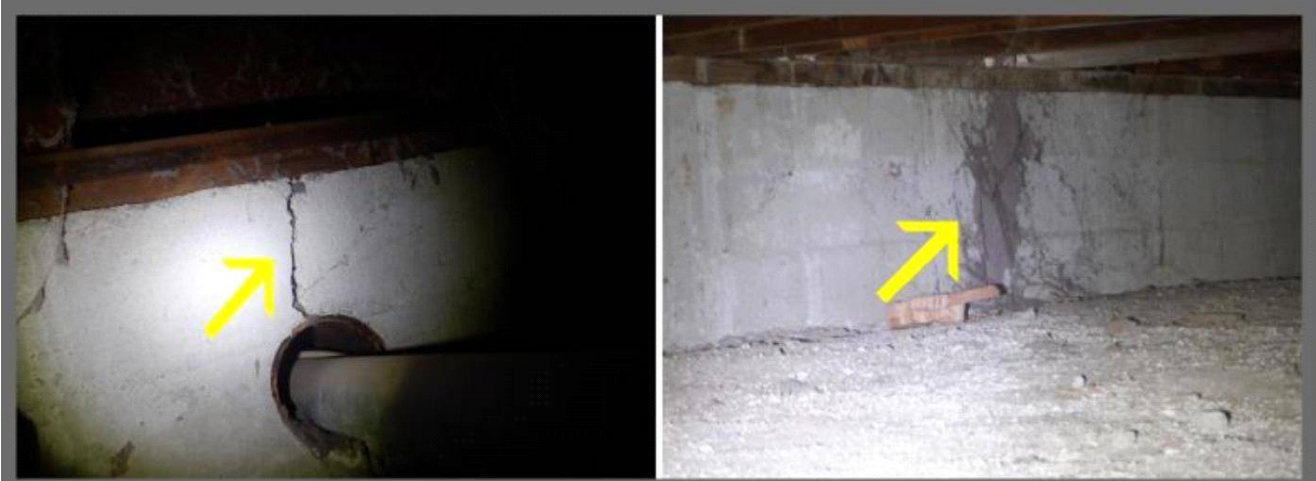
Cracks & patching
