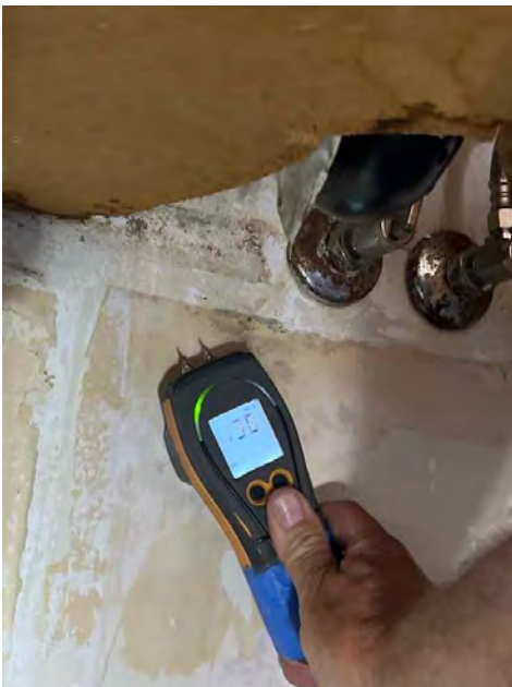
Moisture Meter Dry Reading
