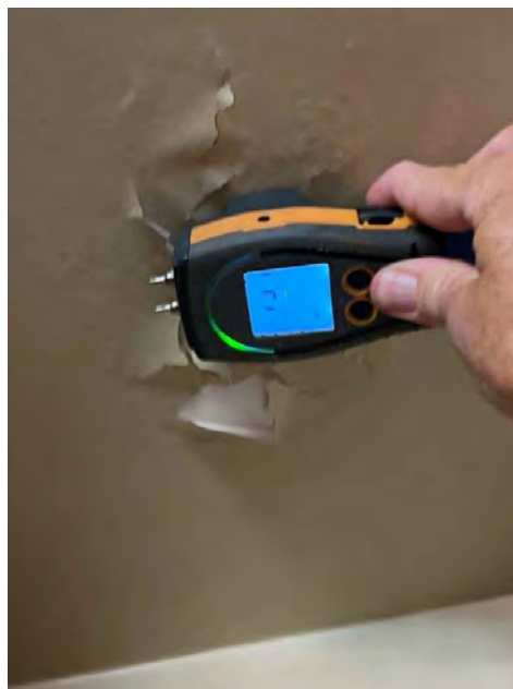
Moisture Meter Dry Reading
