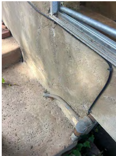
Left exterior walkway
