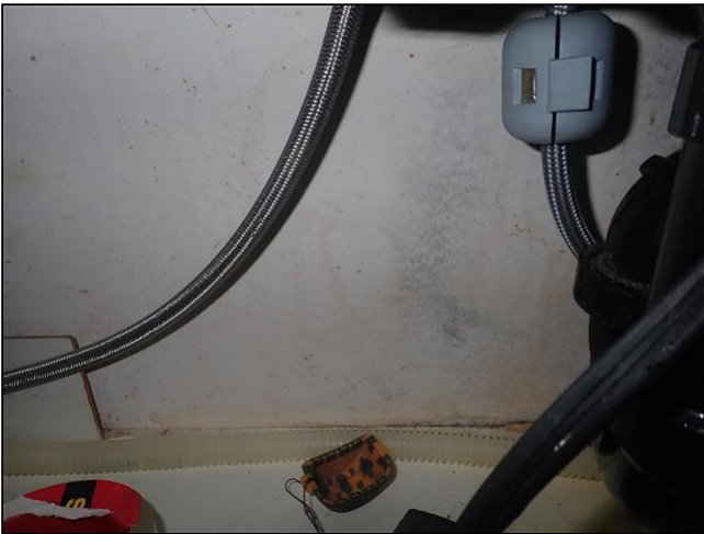
3.2 Item 3(Picture) Under kitchen sink.
