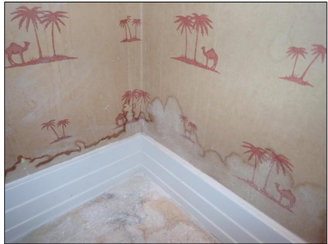
3.2 Item 4(Picture) Half bathroom.
