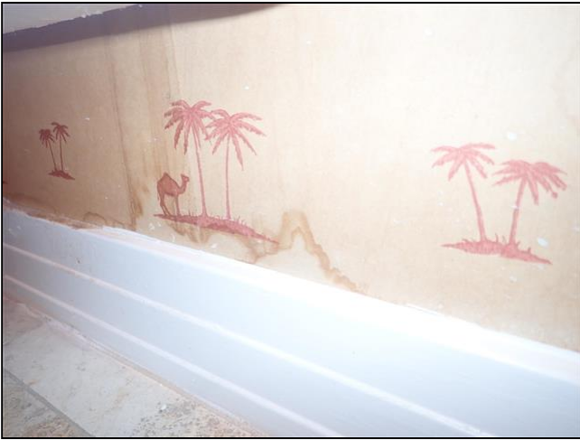
3.2 Item 5(Picture) Half bathroom.
