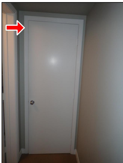
3.6 Item 1(Picture) Master bedroom.
