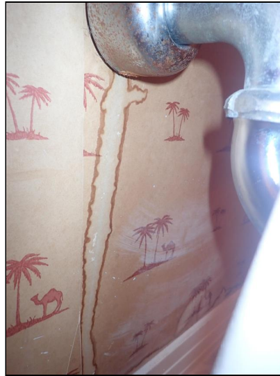
3.2 Item 6(Picture) Half bathroom.
