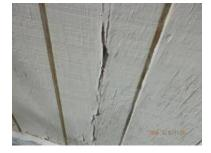
[CR] There were gaps between the wood siding and adjacent materials. These conditions are conducive to moisture intrusion/deterioration. We recommend correcting the condition(s) noted.
