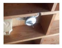
[SC] There was improper wiring installed in the form of nonmetallic sheathed wiring exposed to human contact and/or mechanical damage. We recommend correcting the condition(s) noted.
