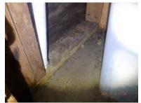
[CR] The insulation (for studio above) was installed upside down. The vapor barrier should be against the conditioned air space. We recommend correcting the condition(s) noted.
