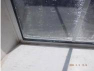
[CR] There was evidence of moisture stains and damage in the window sill(s). The area tested actively wet during the inspection. We recommend locating and correcting the source as well as any damaged materials.
