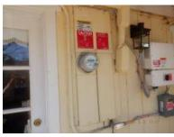
803 SERVICE RATING: 120/240 volt system, rated at 175 amperes.
