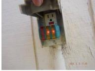
[CR] There was no power at the GFCI receptacle and it would not reset. We recommend correcting the condition(s) noted.
