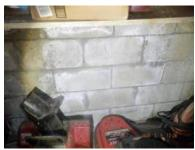
[SC] There were homeowner-built shelves hanging from the ceiling/walls. The additional weight can damage the framing. We recommend it be engineered or removed.
