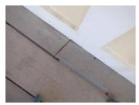
[CR] The deck was located too close too the ground. This condition is conducive to moisture damage and deterioration. We recommend correcting the condition(s) noted.
