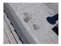
[FE] The shingles had extensive granulation loss, erosion and cracking throughout the shingled surface. These condition(s) are conducive to moisture intrusion, **roof leaks**, and deterioration. We recommend further evaluation and corrections by a specialist in the appropriate trade.
