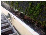
[CR] The rain gutter(s) were improperly sloped and holding water. We recommend correcting the
