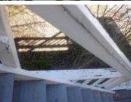
[RU] The guardrail(s) installed were in serviceable condition and appear to have meet the standards at the time of construction, however the wide spaces between the balusters pose a hazard for small children. Modern construction requires a maximum of 4 inch openings. While upgrading is not required, additional measures for child safety like netting or some other means is strongly recommended.
