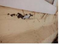
[CR] There was a condition known as efflorescence on portions of the foundation walls. This is a salt deposit left when moisture in the foundation evaporates. It indicates that the foundation is experiencing wet and dry cycles. Efforts should be made to identify the source of the moisture and correct this condition. We recommend the exterior grading and drainage be improved to divert moisture away from the foundation.
