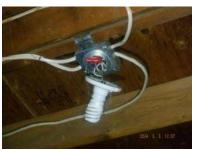
[SC] There was improper wiring in the attic in the form of splices in wiring that were not contained in approved/covered boxes. We recommend correcting the condition(s) noted.
