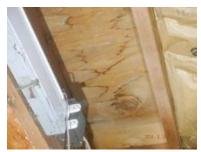
[SC] The garage ceiling/wall tie framing was being used for storage. The additional weight can damage the framing. We recommend it be engineered or removed.
