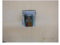
[SC] The GFCI receptacle was providing power, but failed to trip when tested. This condition is safety hazard. We recommend correcting the condition(s) noted.
