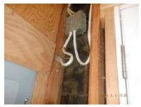
[SC] There was improper wiring installed in the form of open junction boxes. We recommend correcting the condition(s) noted.
