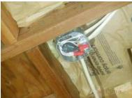
[SC] There was improper wiring installed in the form of improperly terminated wiring. We recommend correcting the condition(s) noted.
