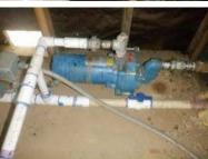
[FE] The well tank was rusted and showed evidence of past leakage. We do not test for function or potable water. We recommend further evaluation and corrections by a specialist in the appropriate trade.
