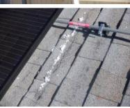
[FE] The shingles had extensive granulation loss, erosion and cracking throughout the shingled surface. These condition(s) are conducive to moisture intrusion, **roof leaks**, and deterioration. We recommend further evaluation and corrections by a specialist in the appropriate trade.
