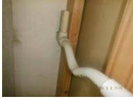
[RU] There was no secondary condensate line installed. We recommend correcting the condition(s) noted.
