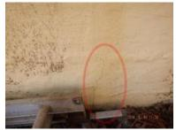
[FE] Horizontal settlement cracks were noted on the interior walls of the finished basement. We recommend further evaluation and corrections by a specialist in the appropriate trade.
