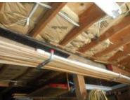
[RU] There was no seismic bracketing at some post to beam connections. We recommend correcting the condition(s) noted.
