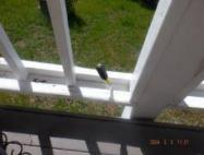
[SC] Some guard rails had large gaps with no balusters. This is a fall hazard. We recommend correcting the condition(s) noted.
