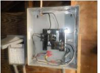
[SC] The neutral wires and the grounding wires were connected to the same busbar. This is an improper wiring arrangement in a subpanel. We recommend correcting the condition(s) noted.
