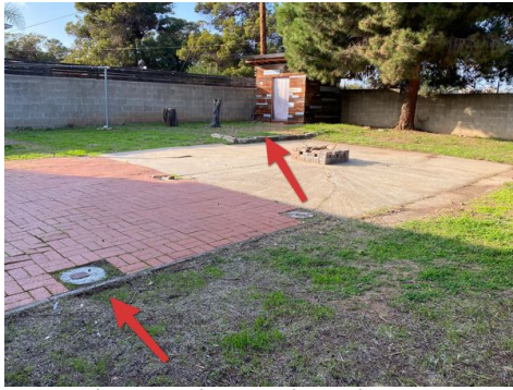
Example Noted at Backyard
