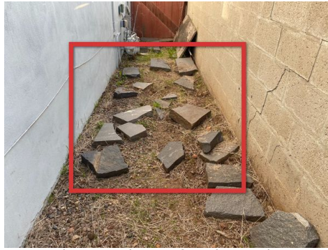
Example Noted at Left Side Yard
