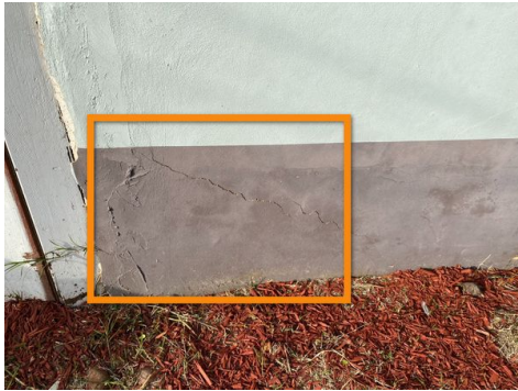
Example Noted at Front Yard
