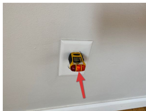
Example Noted at Living Room
