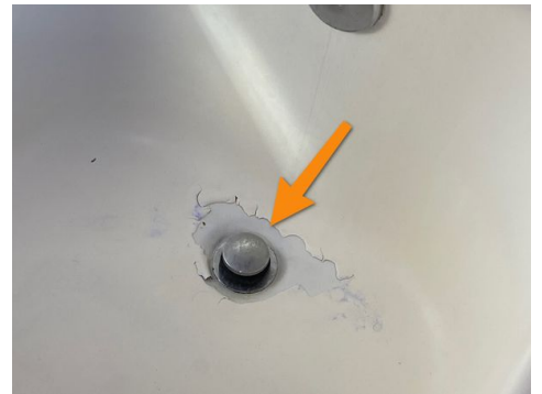
Example Noted at Hall Bathroom
