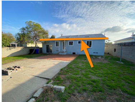
Example Noted at Backyard
