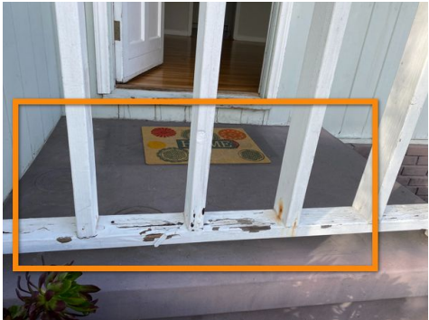
Example Noted at Front Yard
