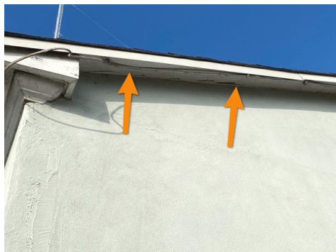
Example Noted at Front Yard
