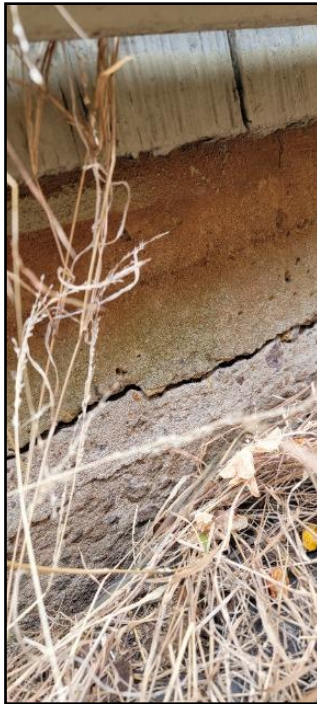
Foundation cracks
