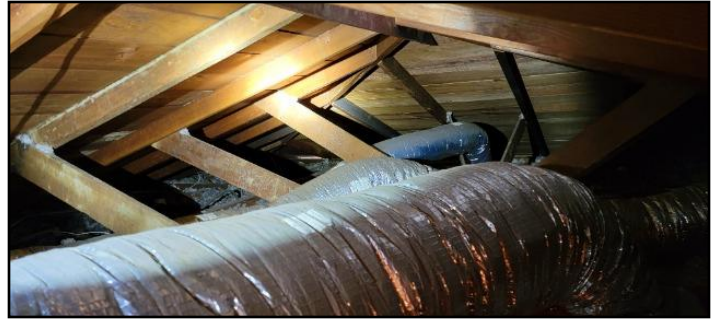
Attic at rear
