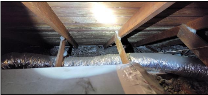
Attic at rear
