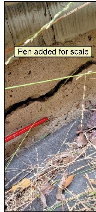
Foundation cracks
