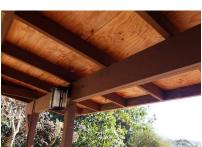
2.44 - There is possible termite and or moisture damage to the front porch and rear patio covers, that should be further evaluated and repaired by a licensed Pest Control Operator.
