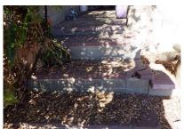
2.52 - There are cracked and or damaged steps at the rear patio. Proper repair by a licensed contractor is advised.
