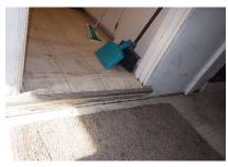
12.5 - A hole has been drilled into the floor, which should be properly repaired.
