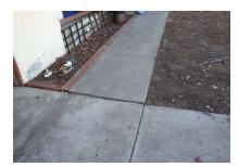
2.28 - The brick style walkways are functional, however, are slightly uneven and or displaced, which may pose as a trip hazard.
