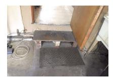
17.10 - The step at the entry to the home is loose and not properly secured, which could be a slip and fall hazard. Further evaluation and repair by a licensed contractor is advised.
