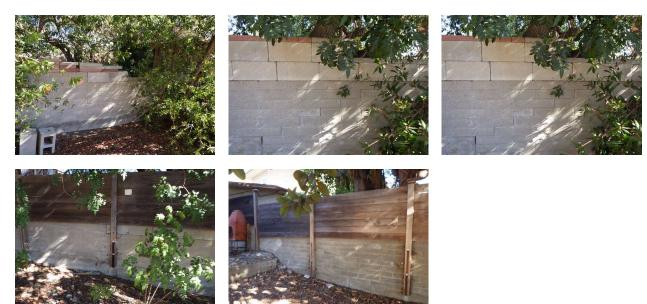
2.32 - There are damaged and or partially removed yard walls noted at the rear of the home. Further evaluation and repair by a licensed masonry contractor is advised.
