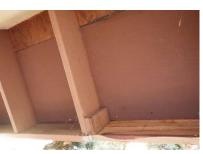
2.38 - There is possible moisture and or termite damage noted in the wood trim, fascia boards, and or eaves at various locations throughout the building. Further evaluation and repair by a licensed Pest Control Operator is advised.
