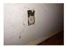
9.17 - One or more cover plates are missing, which should be replaced.
