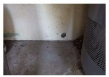
2.20 - There are moisture stains and or damage in the stucco at the base of the walls, at various locations around the home. This is a cosmetic defect which is caused by poorly aimed sprinklers, roof run-off, and or improper soil height. Further evaluation and repair by a licensed contractor is advised.
