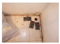
12.6 - There are patched and or damaged areas in the floor under the refrigerator, which you should question the seller about, or have further evaluated by a licensed contractor.
