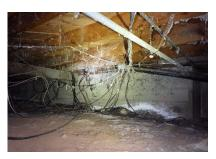
1.11 - The crawl space is contaminated by rodents, which is a significant health hazard, and should be evaluated by an exterminator as soon as possible. Rodents can compromise not only the crawlspace and its various components, such as ducts and insulation, but can eventually contaminate the living space as well. Consequently, we disclaim any further responsibility for evaluating the crawlspace and its components.
