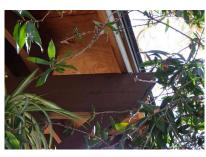
2.45 - There are moisture stains and signs of prior leakage on the underside of the rear wood patio cover. Further evaluation and repair by a licensed roofer is advised.
