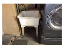
16.6 - The sink drains too slowly, and should be serviced to ensure that the blockage has not progressed beyond the trap.
