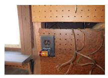
17.16 - There is exposed Romex wiring noted on the walls and or ceiling of the garage. Further evaluation and repair by a licensed electrician is advised.
