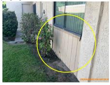
Damaged stucco noted under patio door(s). Builders stucco's the slab for looks, but the stucco has no wiring to help it bond. All slabs will wick moisture and the moisture will caused the stucco to peel. Recommend area be covered with metal.
