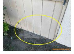
NR It appears that sprinklers are spraying against house, adjustment needed to sprinklers at rear and right side
