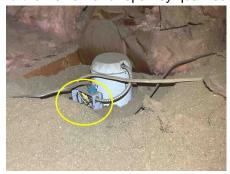
Recessed lights in attic are covered with insulation, inspector could not verify if lights are non-IC rated, recommend verifying if lights are IC rated for contact with insulation. Non-IC rated lights require at least 3 inches clearance to combustibles
