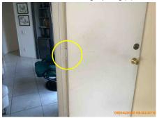
Door from garage to interior of the house is required to be weather stripped and have proper threshold and a bottom sweep installed
