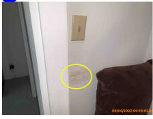
Possible asbestos containing material in closet ceilings, We recommend further review and repairs by a qualified specialist in the appropriate trade.
