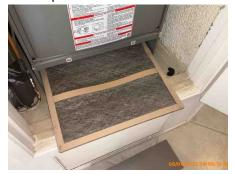
RM Heater filter is dirty, new filter is needed, suggest cleaning/changing filter regularly
