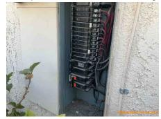
Missing protective bushing for wires that enter inside the main electrical panel, wire should be protected from metal enclosure. Recommend further review and repair by qualified Electrical Contractor.
