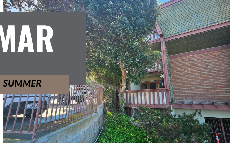
In anticipation of scaffolding being installed, the tree to the left of the parking garage entrance will be removed.
