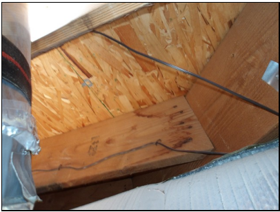
master bedroom attic
