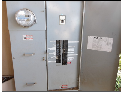
Electric front exterior
